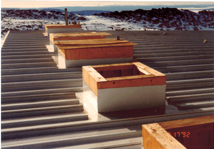
Figure 3: Constructing roof hatches for a variety of remote sensing instruments.
