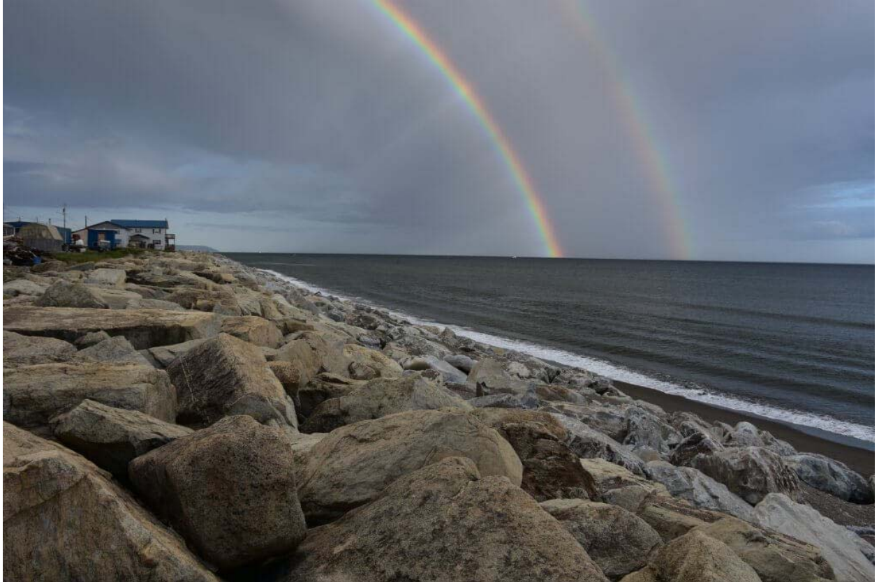
Photo 1: Seawall in Nome, Alaska. An example of a structural adaptation. Photo courtesy of S. Jeff Birchall, taken August 12, 2016, 1am.
