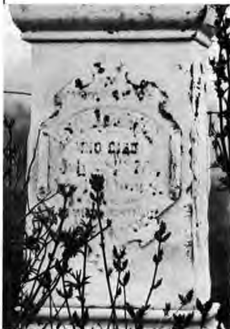
CARBONIC ACID IN RAIN OVER A PERIOD OF 109 YEARS has attacked the calcite in a marble tombstone and made the inscription almost illegible.
