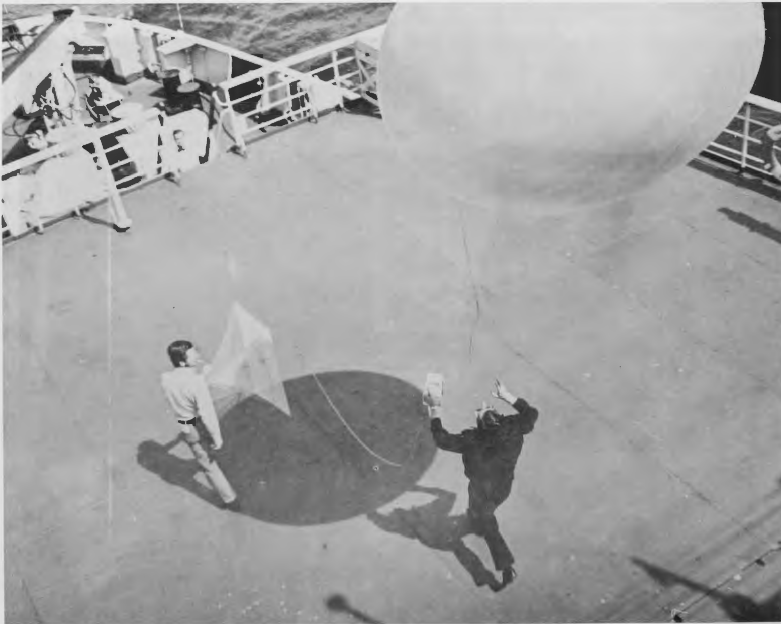
Figure 3. Launching the radiosonde balloon for an upper air observation.
