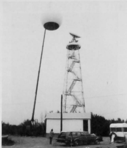
Radome being installed at Britt, Ont.
