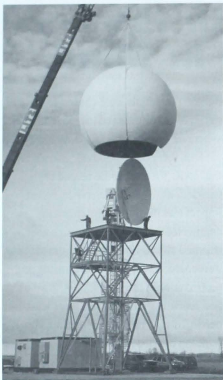
The Woodlands Doppler radar under construction.
