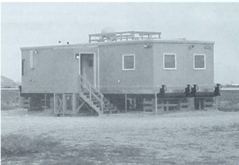
The new weather station in Churchill, Manitoba, was designed with the environment in mind.
